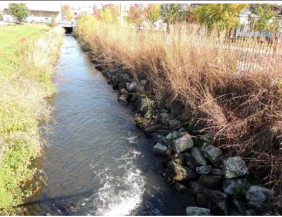
Streambank Stabilization
